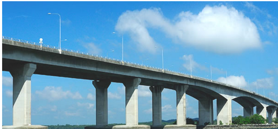
Malaysia-Singapore Second Link Bridge
