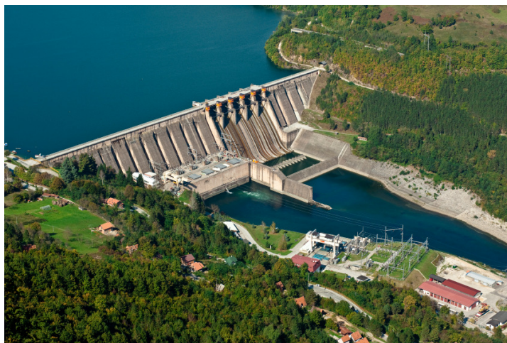
Hydroelectric Dam: This dam in Serbia uses instrumentation to monitor its structural stability
