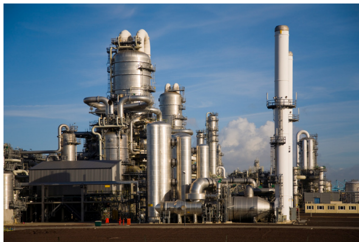
Oil Refinery: Connects to SAGD wells via long pipelines. There are many places within one of these refineries to use dataTaker products.
